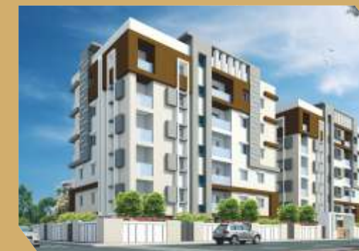
Sri Tirumala Hamilton @ Padmarao Nagar
