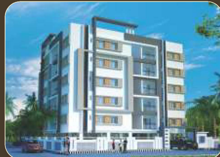
Sri Tirumala Lotus @ Sivarampally
